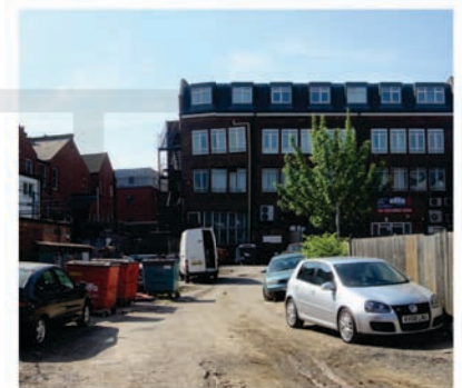
Fig. 6.49: Looking southward into existing site, currently as service yard serving properties along College, Station and St Anns Road.
