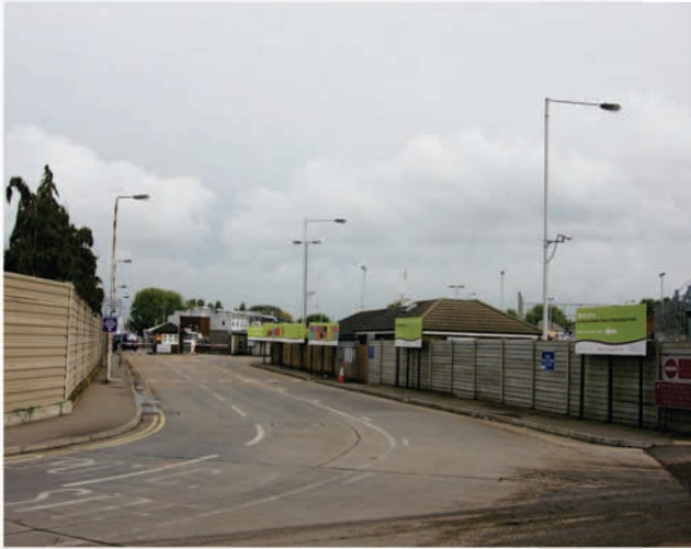
Fig. 6.26: Existing site approached along Forward Drive.
