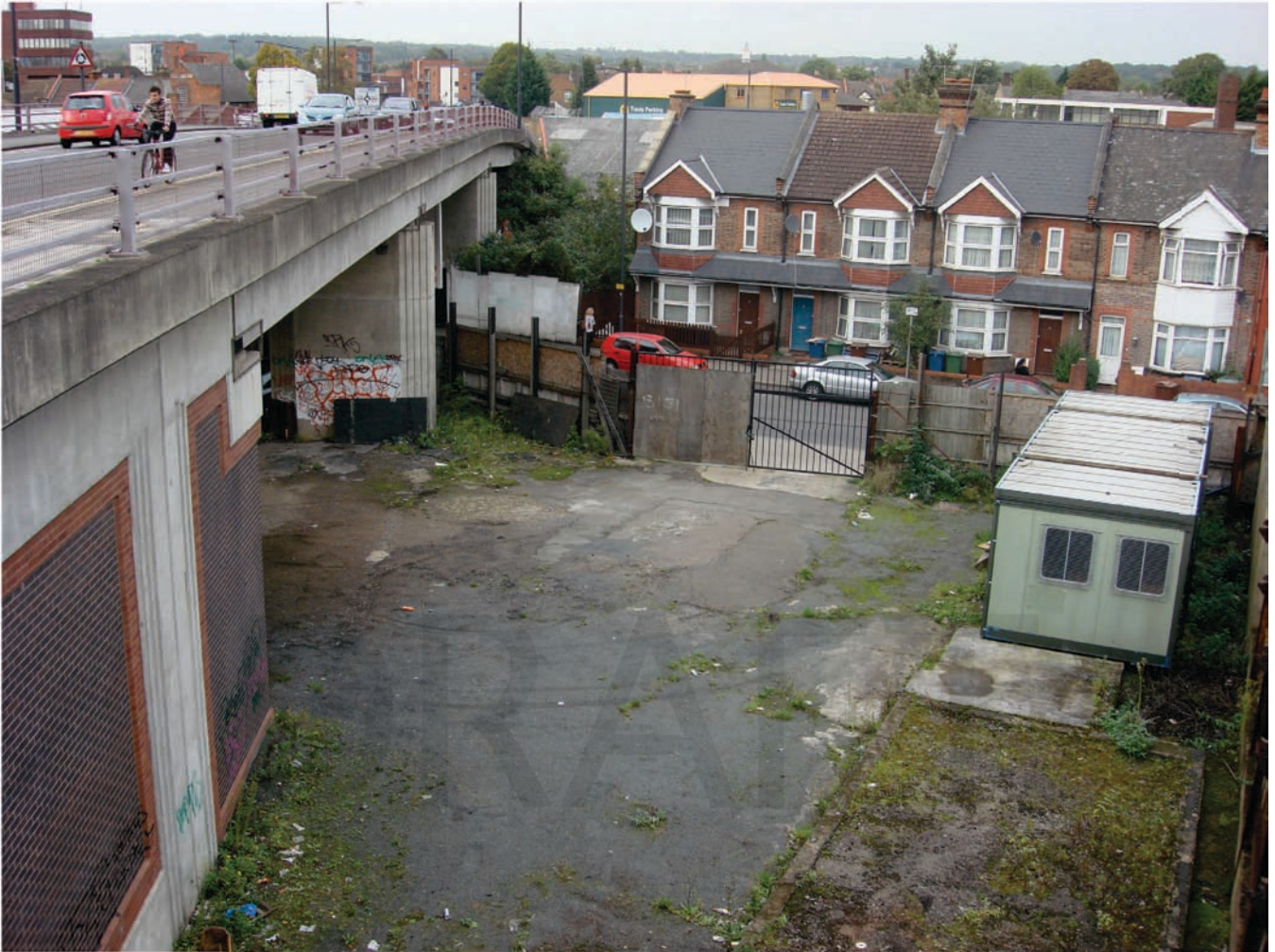
Fig. 6.20: Example of existing Palmerston Road/George Gange Way site.
