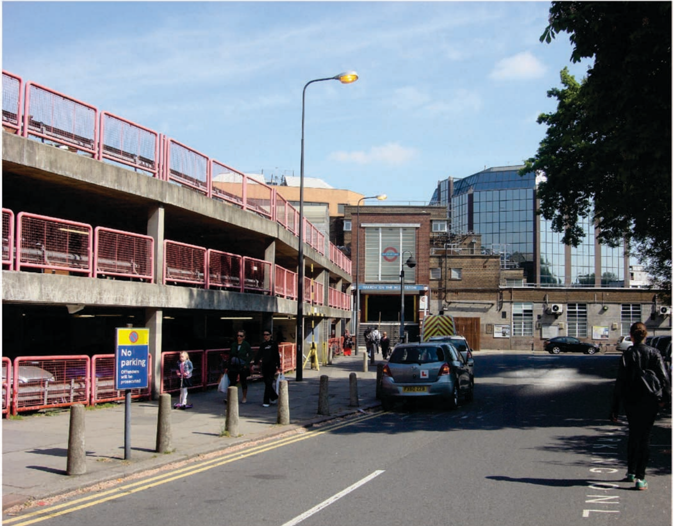
Fig. 6.53: Existing site looking north toward Harrow on the Hill station's southern entrance.
