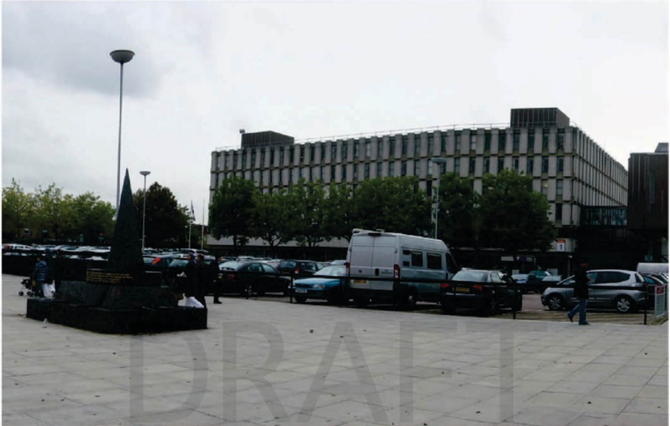
Fig. 6.30: Looking west toward Civic One from Station Road with the war memorial in the foreground.
