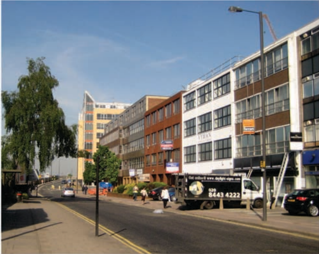
Fig. 6.45: Existing site looking west along College Road.
